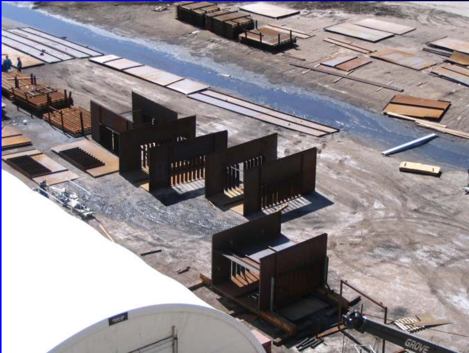
Pre-Assembly of Inlet Plenum Sections
