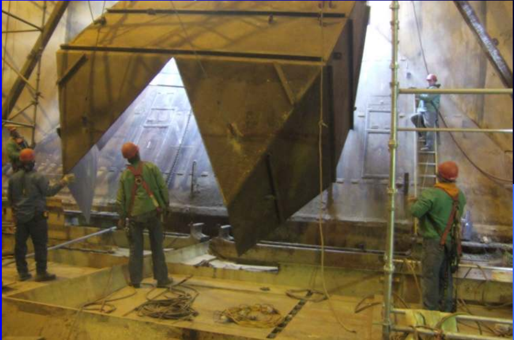
Inlet Nozzle Transition Being Lowered into Place
