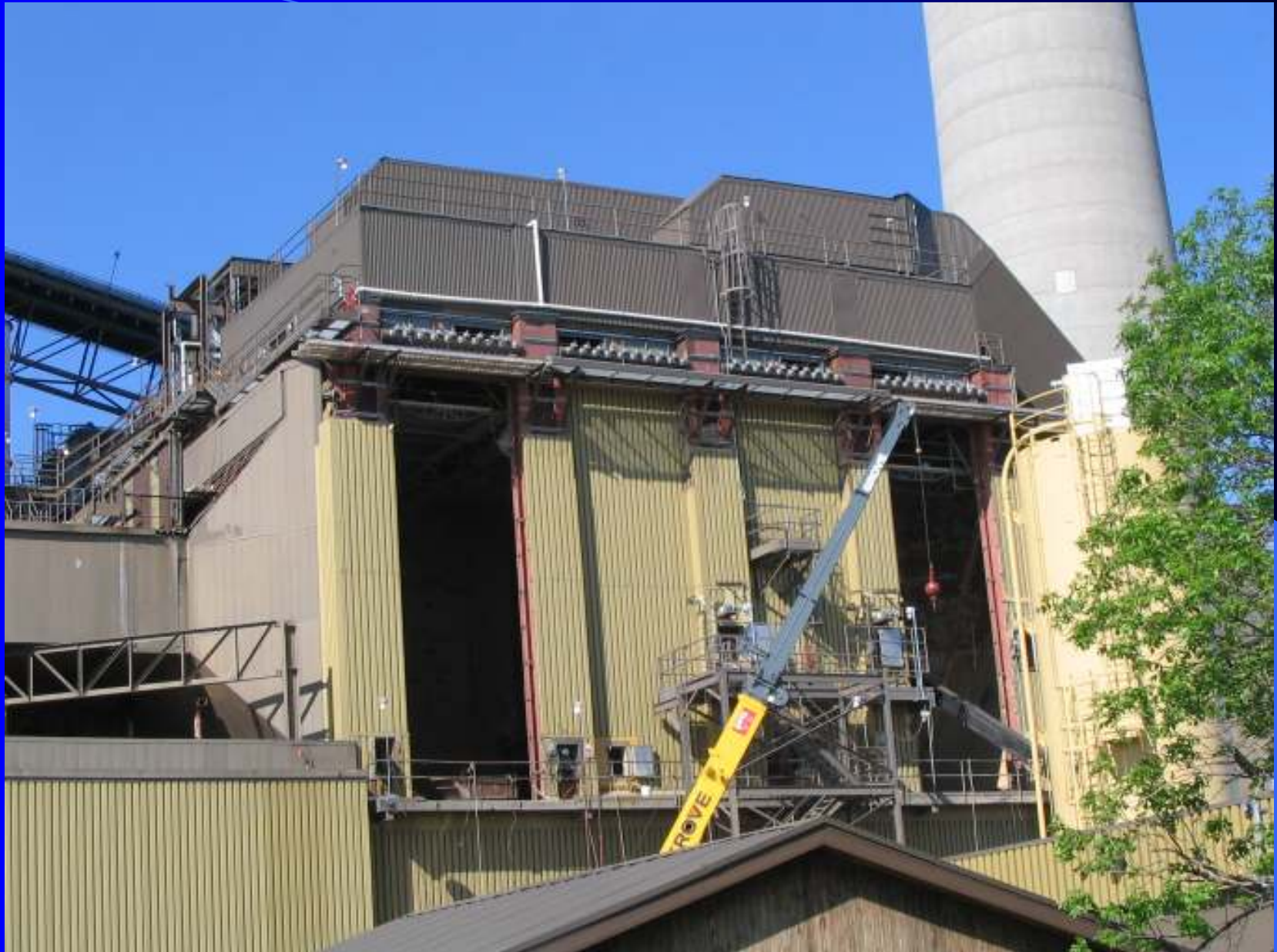
ESP Side Cut-outs for AHPC Demolition
