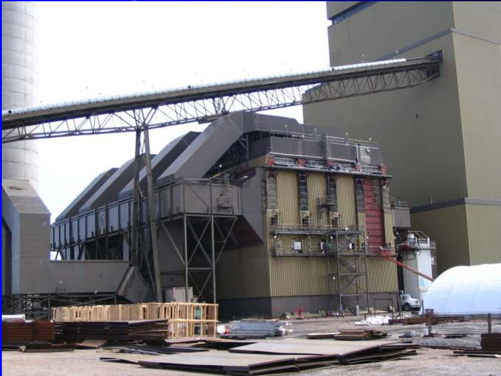
Big Stone ESP – Four Chambers
