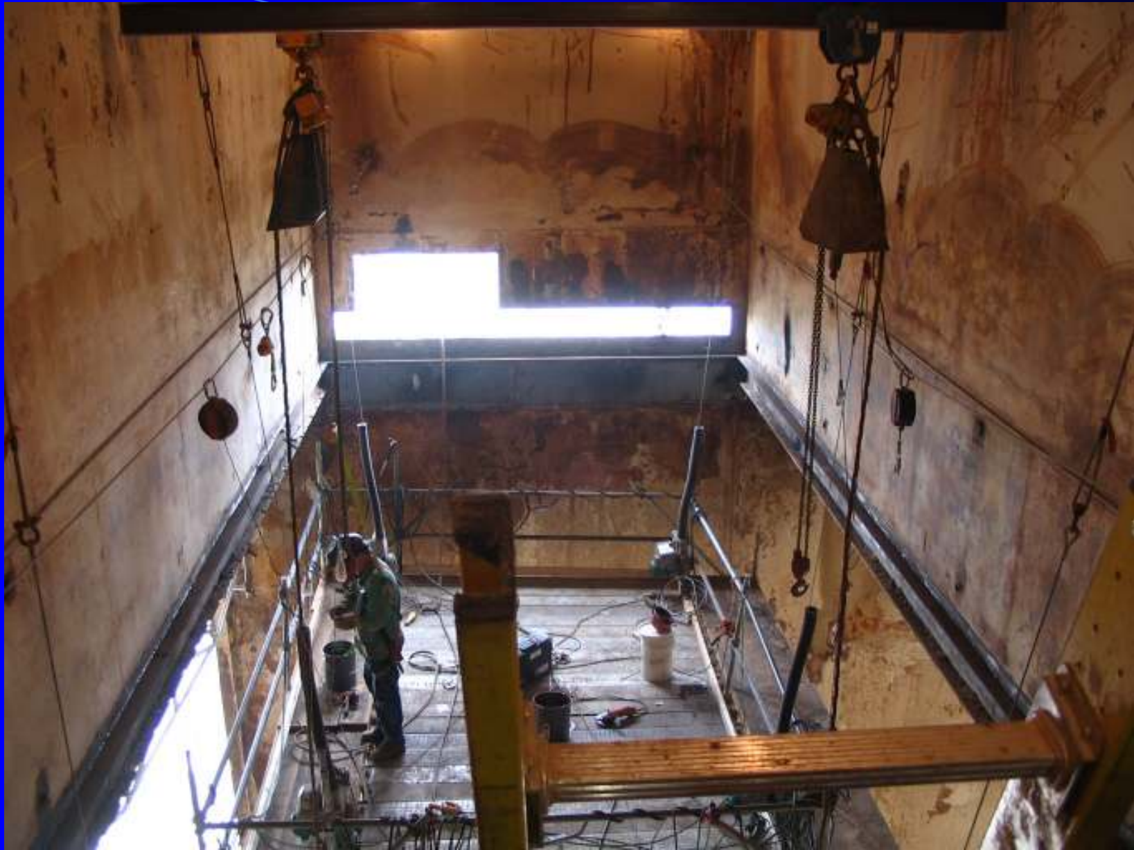
Compartment Tubesheet Shelf Installation
